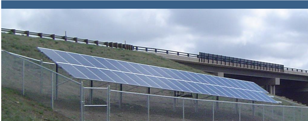
Solar site on the NWP Right-of-Way slope.
